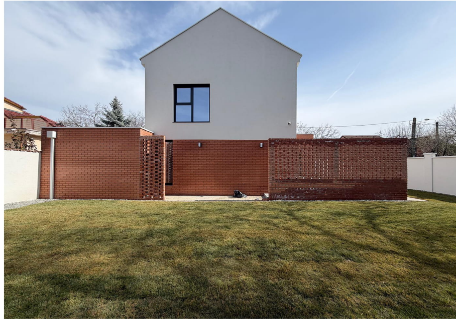
FATADA POSTERIOARA/ REAR FACADE
